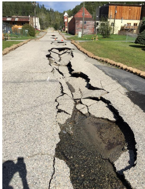
Greenwood Street Culvert Failure (May 2017)
